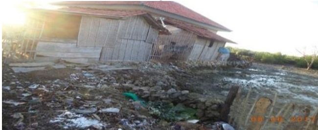
Fig. 4. Coral reefs have become the Foundation of a building
