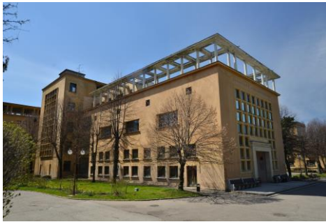
Fig. 4. Main Building No.1. Entrance Group and Concert Hall (current state).
