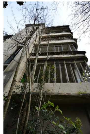
Fig. 2. Main façade element of the health resort in Sochi (current state).
