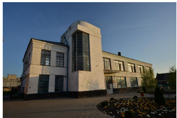
Fig. 5. The factory kitchen in Tikhoretsk (current state).
