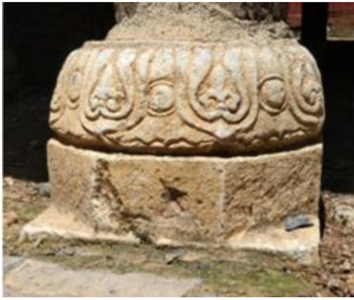
Fig. 5. Tub-covering type plinth (the Tan ancestral temple).
