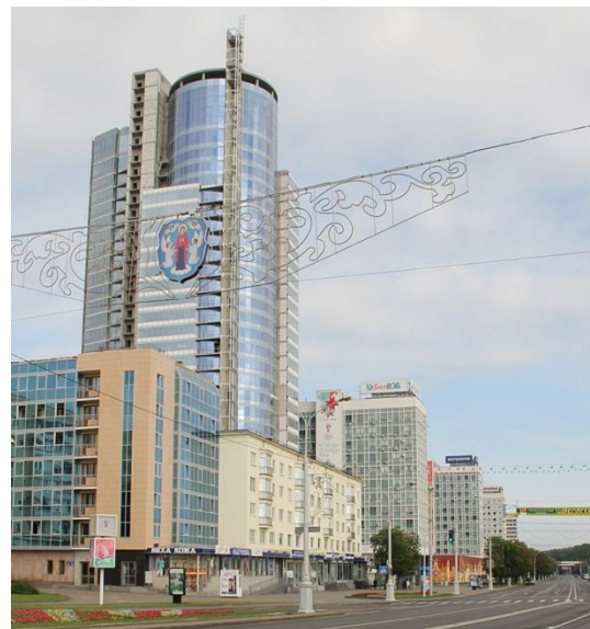
Fig. 5. Violation of ensemble. Minsk.
