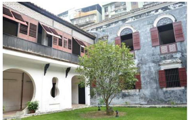
Fig. 7. The Square Inner Courtyard.
