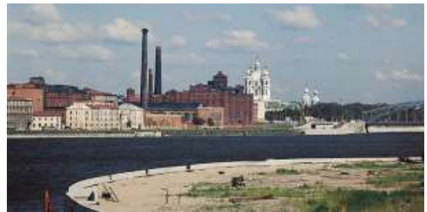
Fig. 5. Panorama of the Nevskaia manufacture before reconstruction work.
