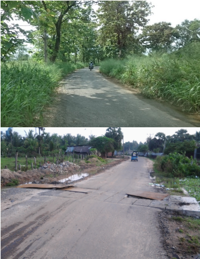
Fig. 2. Limited shoulder width and lack of proper highway structures
