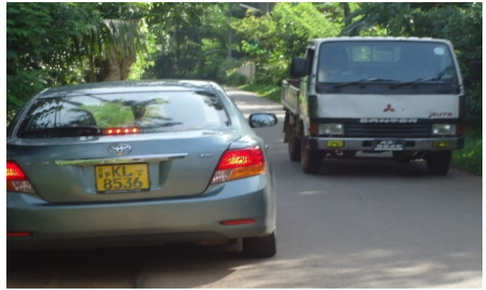
Fig. 1. Limited provision of passing bays and low carriageway width
