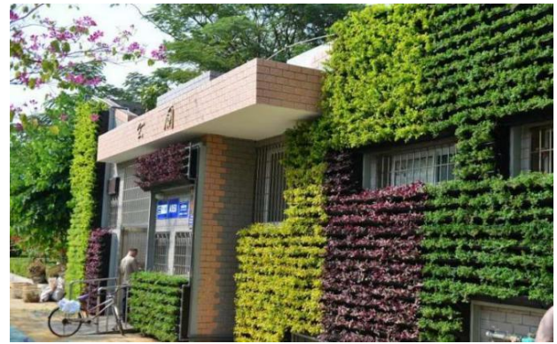
Fig. 5. Plant vine on facades of outer walls.
