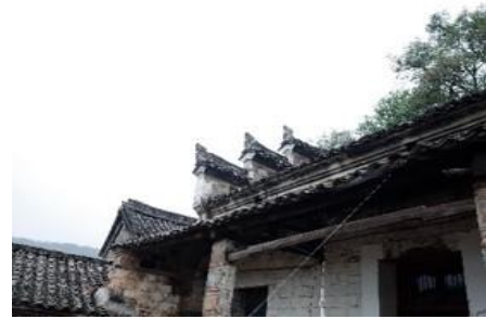
Fig. 7. Photograph of partial roof (author's self-photograph).
