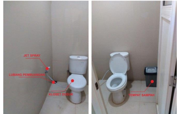
Fig. 5. Cubical Toilet Seats (source: Author's Documentation)
