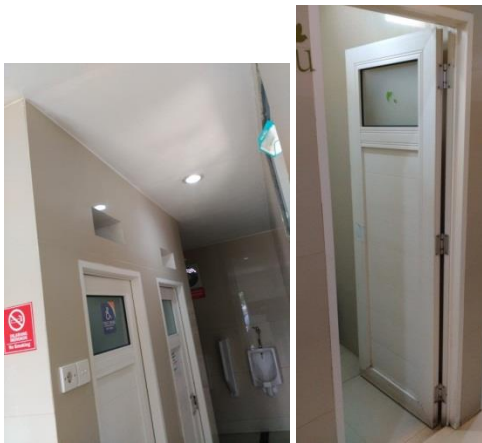
Fig. 3. Toilet Door (Source: Author's Documentation)
