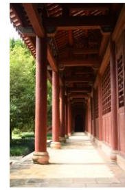
Fig. 6. Corridor of East-west verandas.
