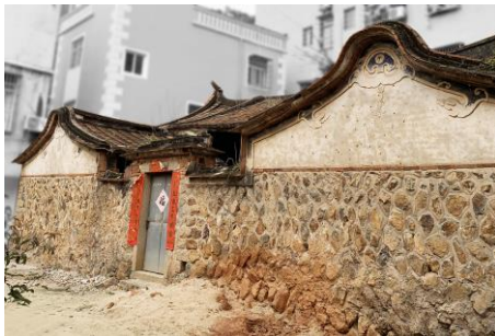
Fig. 4. Traditional residential buildings in South Fujian.
