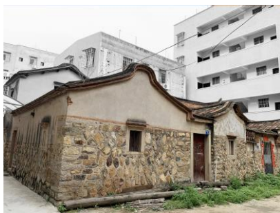
Fig. 5. Traditional residential buildings in South Fujian.
