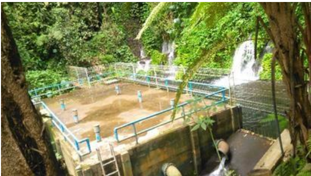
Fig 4. Water Reservoir in Sumberpitu Water Springs
