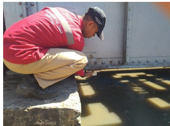
Fig. 4. Installation of Device at BH 82.
