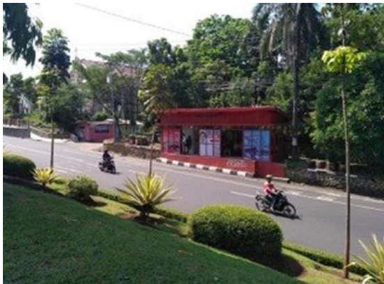
Fig. 6. Bus stop condition Elizabeth.
