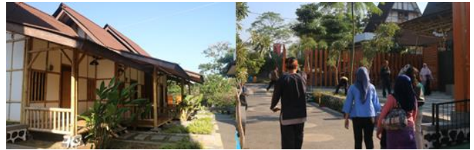
Fig. 5. Building and visitors activity in Cibiru cultural house.
