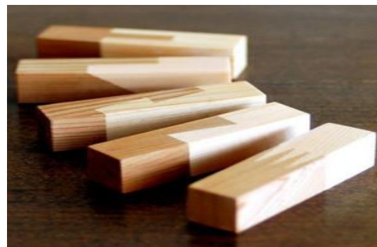
Fig. 6. Tenon-and-mortise structure 1.
