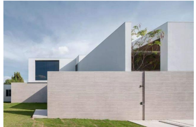
Fig. 3. A modern building clad in ceramic tiles.
