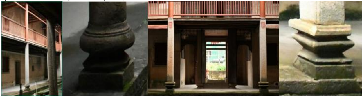
Fig. 2. Plinth and pillars of the Zoumalou, plinth and pillars of the hall.
