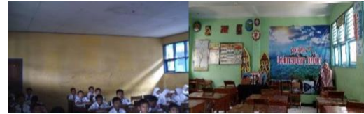
Figure 2. School condition after development of PPK-BKLMK
