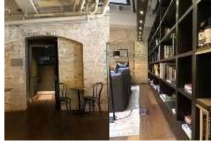
Figure 11: Timber flooring at 1 st storey
