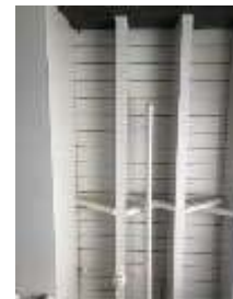
Figure 12: Exposed Timber Ceiling Floor Structure
