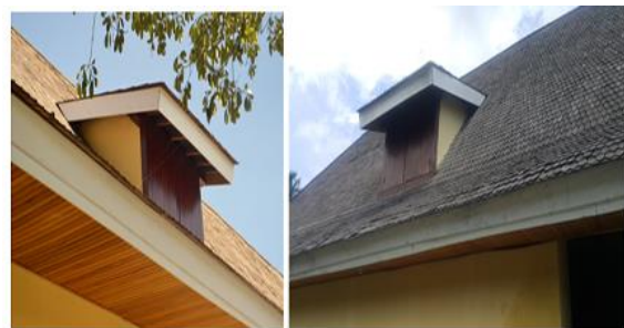
Figure 3 Dormer roof of armory warehouse
