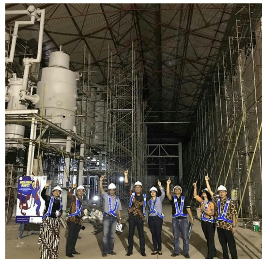
Figure 3 "De Tjolomadoe" during construction
