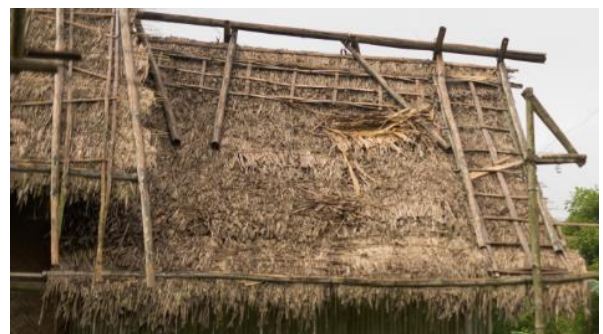
Figure 5 The tobacco barn roof with the reinforcement structure ( cecek )
