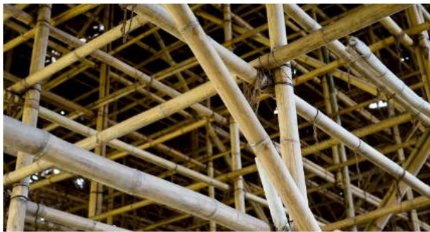
Figure 7 Bamboo structure of Gudang Atag
