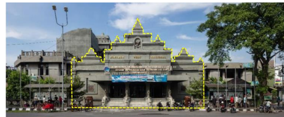
Figure 2 The facade of the cultural heritage building.
