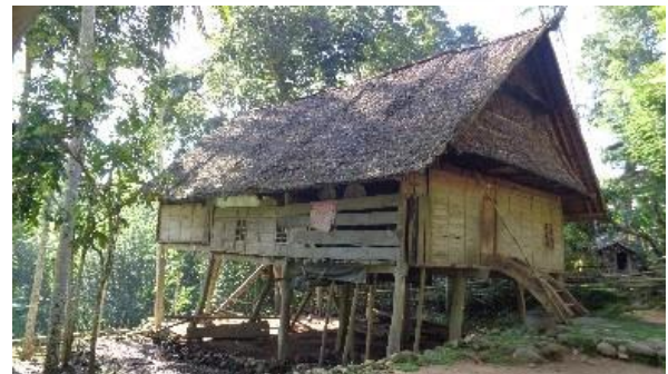
Figure 6 Curved Piles on Traditional Ammatoan Houses
