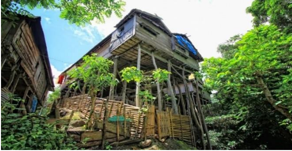
Figure 7 Tall Piles in a Traditional Bitombang House
