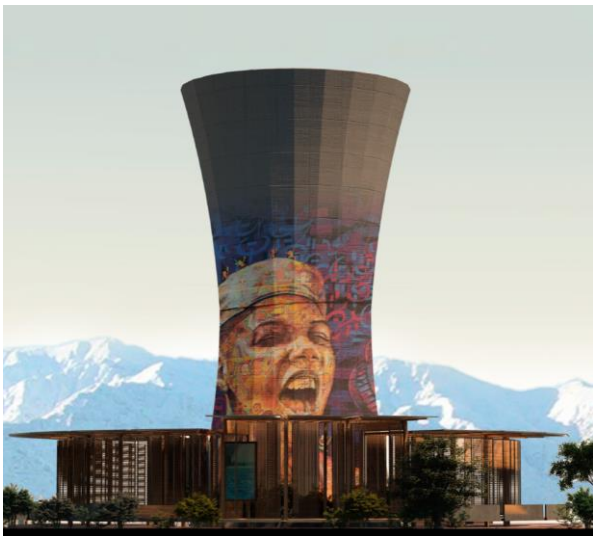
Figure 14. High social impact project in operative water tanks. New social landscape in Santiago de Chile.
