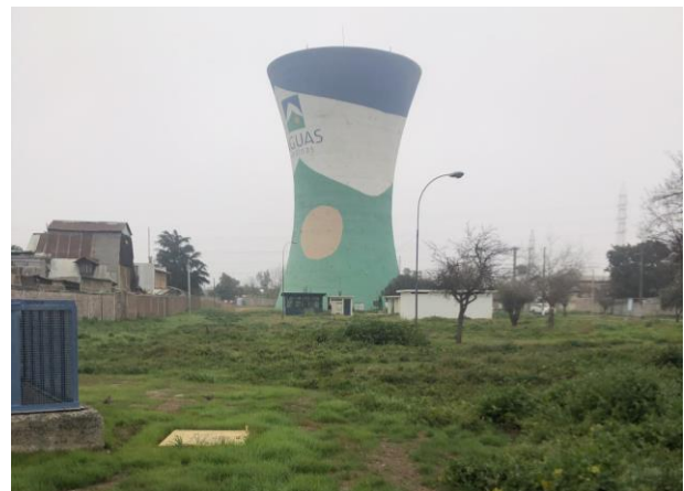
Figure 9. Existing landscape inside operative drinking water infrastructure in Chile
