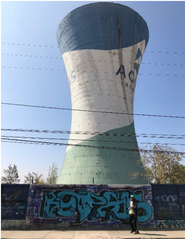
Figure 8. Walled water tank in a low-income area in Chile.
