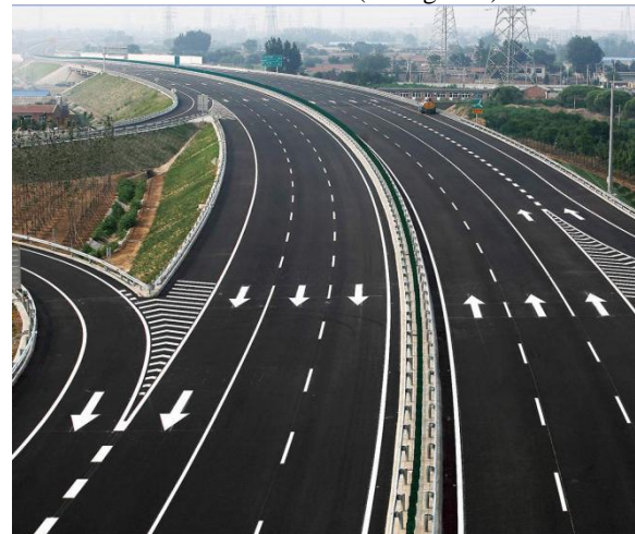
Figure 1. The smoothness of Expressway Pavement
