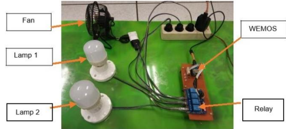
Figure 6. Implementation to the plant
