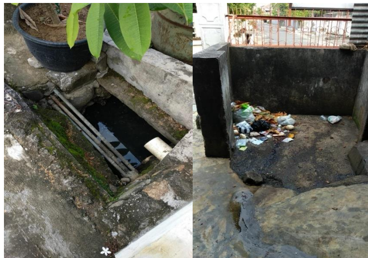
Figure 3. The sewer and the trash place
