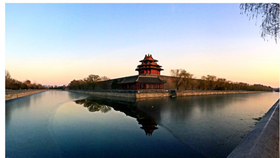
Figure 1 The corner building of the Forbidden City
