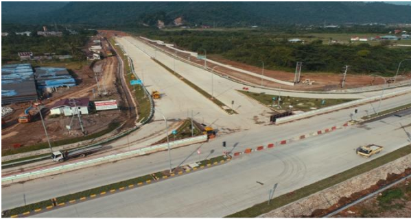
Figure 2. Toll Road of Padang- Sicincin
