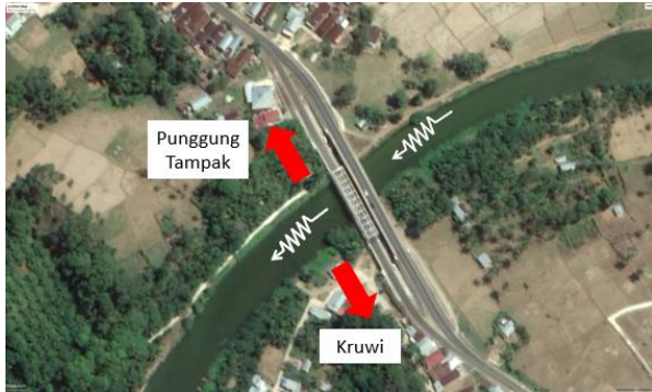
Figure 3 Aerial Photo of Way Pedada Bridge
