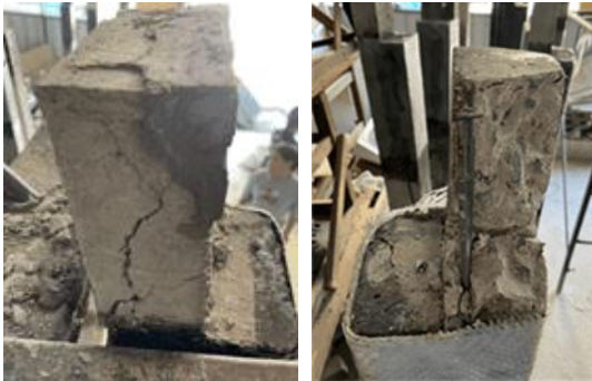
Fig. 6. Failure of repaired columns using CFRP laminates (left) and GFRP laminates (right).
