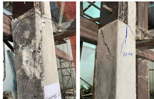
Fig. 4. Failure of control specimen (left) and pre-cracked column for FRP repair application (right).
