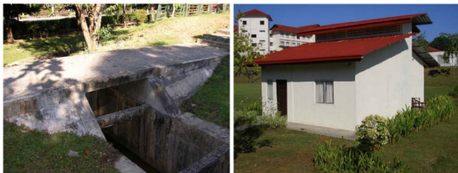
Fig. 5. Oil palm shell concrete used in a footbridge and a small house [14].
