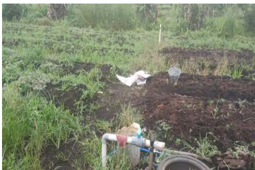
Figure 1 Drilling Well Located on Community-Owned Land Community
