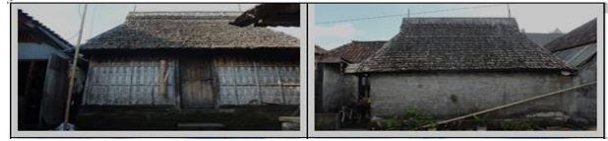
Figure 3. Documentation of Umah Paon in Penglipuran Village
