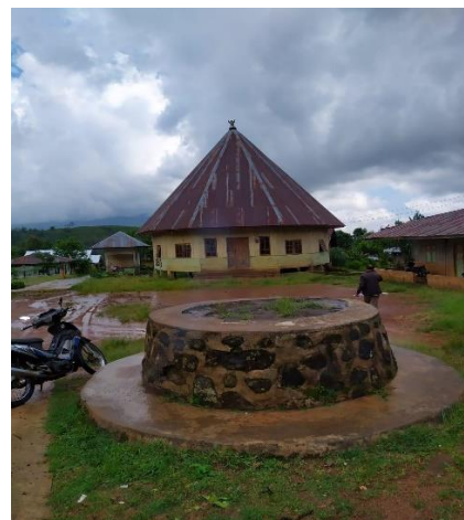
Fig. 3. Outside view of Meler village traditional house.
