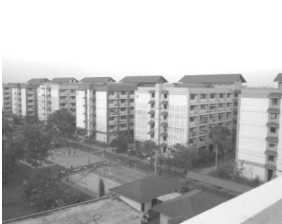
FIGURE 1: Rusunawa RGTC with sports facilities (Source: UPRS Cakung Barat).
