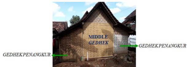
Figure 4. Using's House Walls
