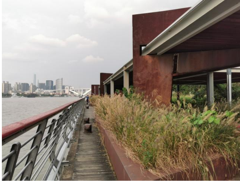
Figure 2 Old wharf after renovation
