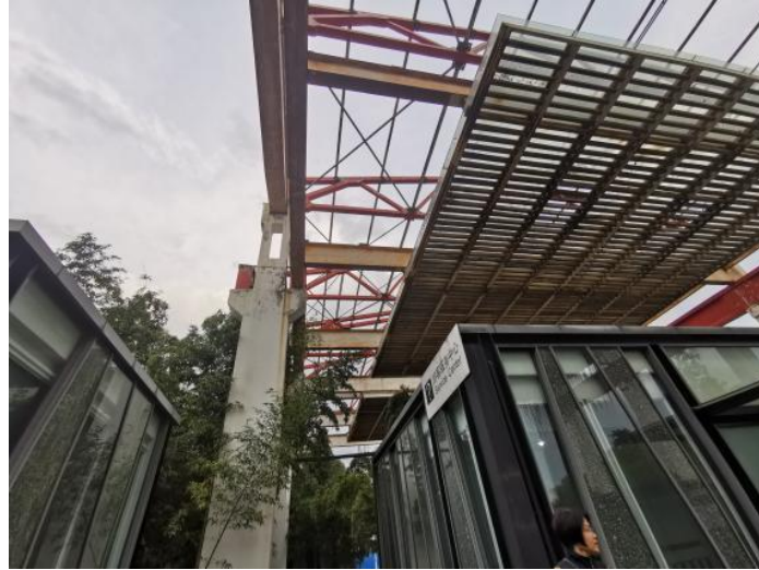
Figure 1 Old factory building after renovation
