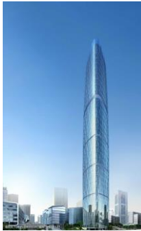
Figure 1 Guangzhou west towe.
