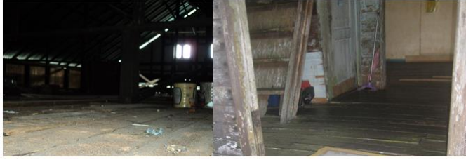
Fig. 2. Powder beetles, fungi, and molds attacks on the stair and attic floor of West Kalimantan's traditional house (the picture taken to the houses in Sambas Town).
