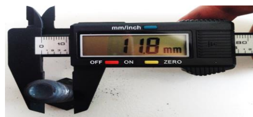
Figure 12 Bolt Diameter Reduction Measurements
