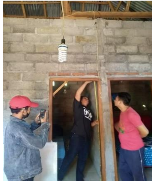
Figure 3 Repairing Guest Room
