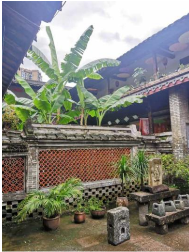
Figure 2 The restored Zhunxing Building.
