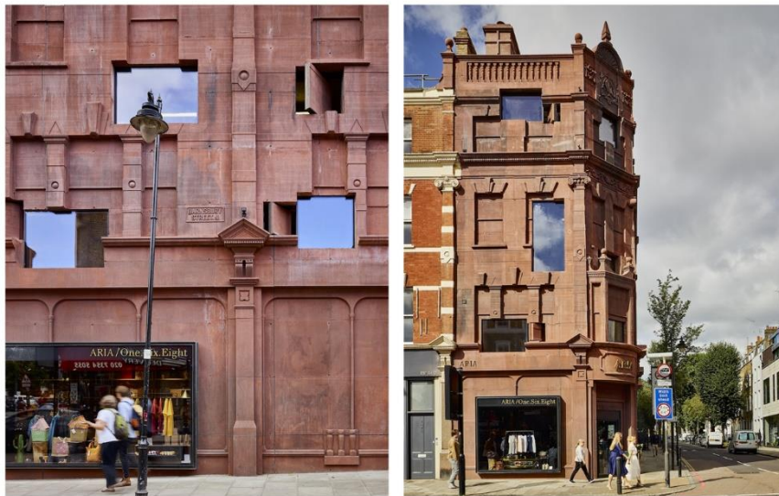
Figure 6 168 Upper Street, London, by Amin Taha + Groupwork, 2017.
