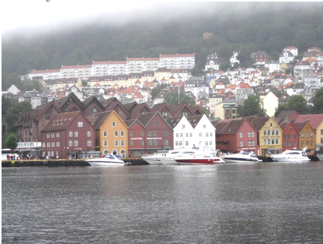
Figure 1 Hanseatic Embankment in Bergen.
