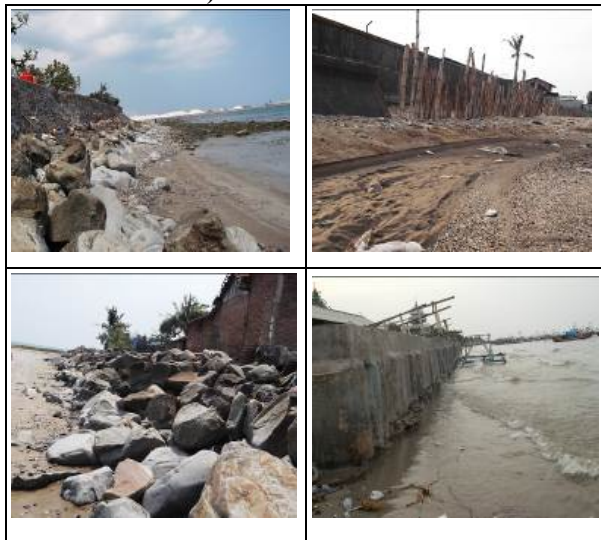
Figure 2. Seawall on preventing abrasion independently built by society (taken on September 8 th 2019)
