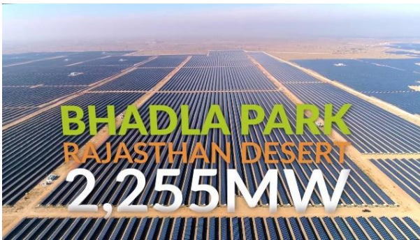
Figure 3. Bhadla Solar Park India: The largest solar park in the world. Source: Asia Record Institute (2020)
